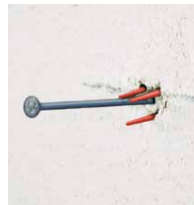
Elastic "stubs" for securing the surveyed measurements are securely marked until after plastering work.
