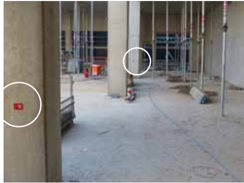
RS30r in industrial construction: Documentation of heights and axis in one product
