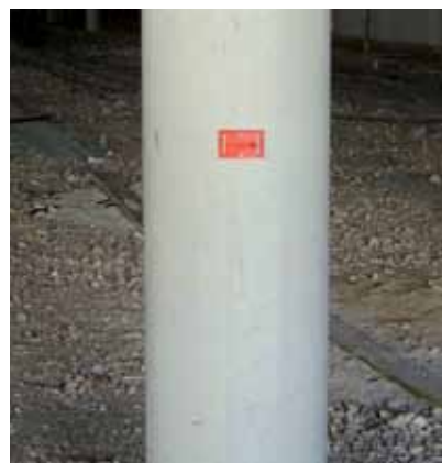
RS21r on a column. The protrusion is cut in 4 - 5 times with a cutter.
