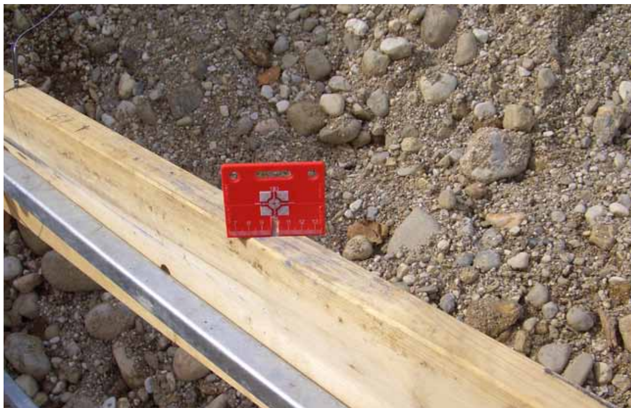
RS95 – Stake-out at the batter board
