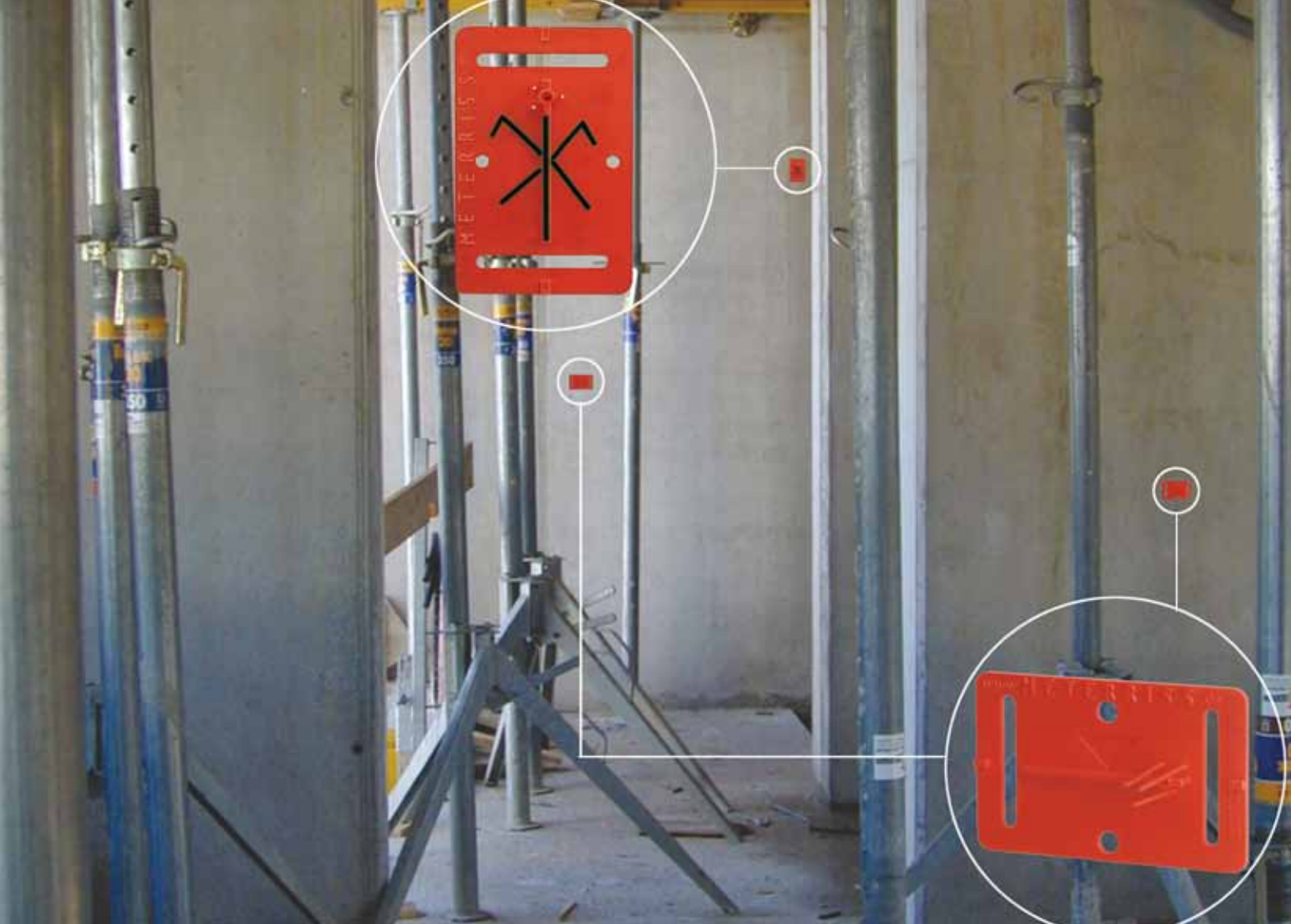
For plastering construction sites and to secure finished floor level (FFL) and axis.
