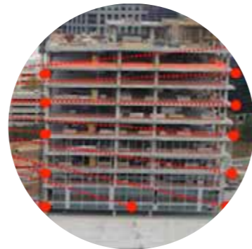
Robotic Total Station Layout
