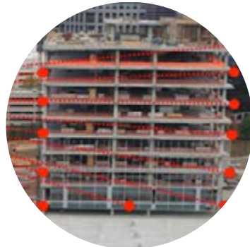
Robotic Total Station Layout
