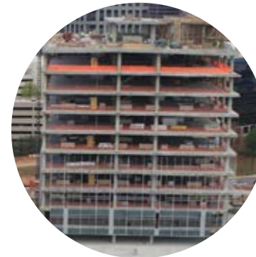
Reality Capture During Construction
